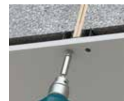
Dry wall bit assembly
